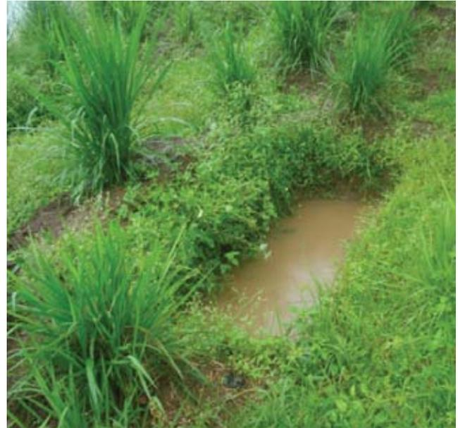
**Image 3: Trenches to trap the runoff rainwater in Namthang block, South Sikkim**
