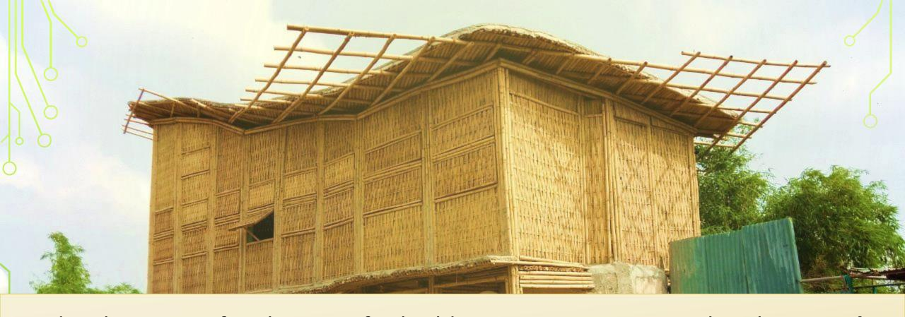
For development of techniques for building construction using bamboo as a **low cost high strength housing material**, an MoU has been entered into with the school of planning architecture (SPA), Bhopal to adapt the vernacular systems of architecture to modern, contemporary applications. Under this, a bamboo lab is being established at SPA bhopal, to research, experiment, and design pragmatic models of bamboo products and buildings.
