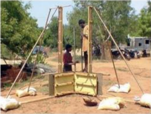
Ramming a corner wall in the first form
