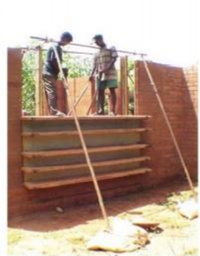
Ramming a long wall in the second form
