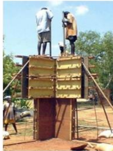
Ramming the fourth form of a corner wall
