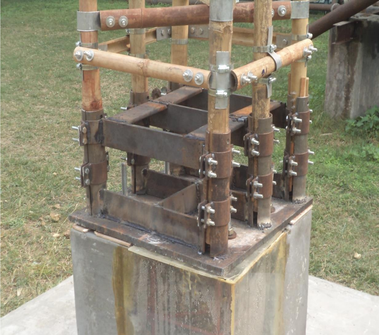
Connection to concrete pedestal
