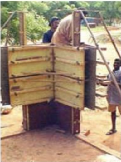
Adjust panels of the third form of a corner wall
