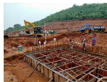
Figure 9: A plant under construction in Odisha
