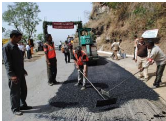
Image 3: Use of plastic waste in road construction
