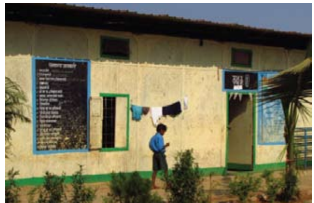
Image 2 and 3: The Kasoli Pota Cabin in Dantewada district, which was the first Pota Cabin constructed under this initiative
