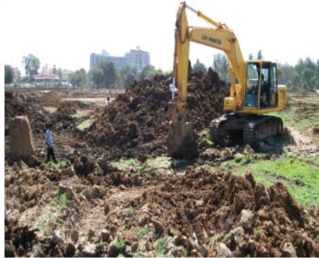
Image 2: Restoration work on Kaikondrahalli lake
