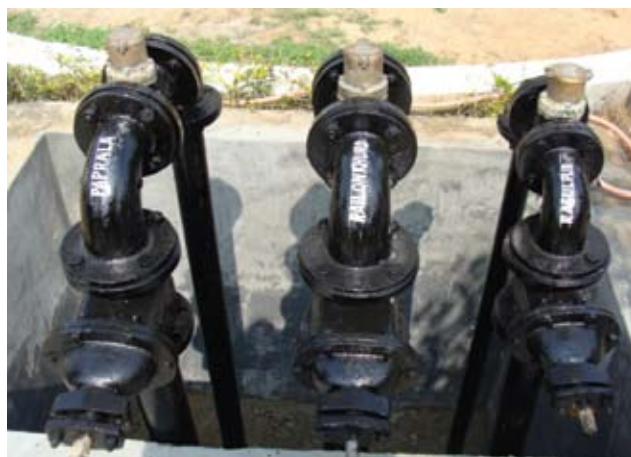
Image 2: Bulk meters set up near the OTR for Paprala, Railon Khurd and Rasalpur villages
