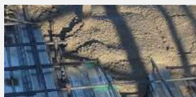
Carbon capture to concrete by Blue Planet
